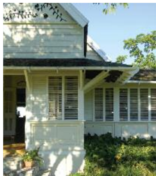
Above: Casa de Velásquez, Santiago de Cuba. Many of the gallery's screen panels are designed to pivot. They offer protection from the sun as well as allowing air to circulate. Photo by Brent Winebrenner. Courtesy of Dr. Michael Connors.
