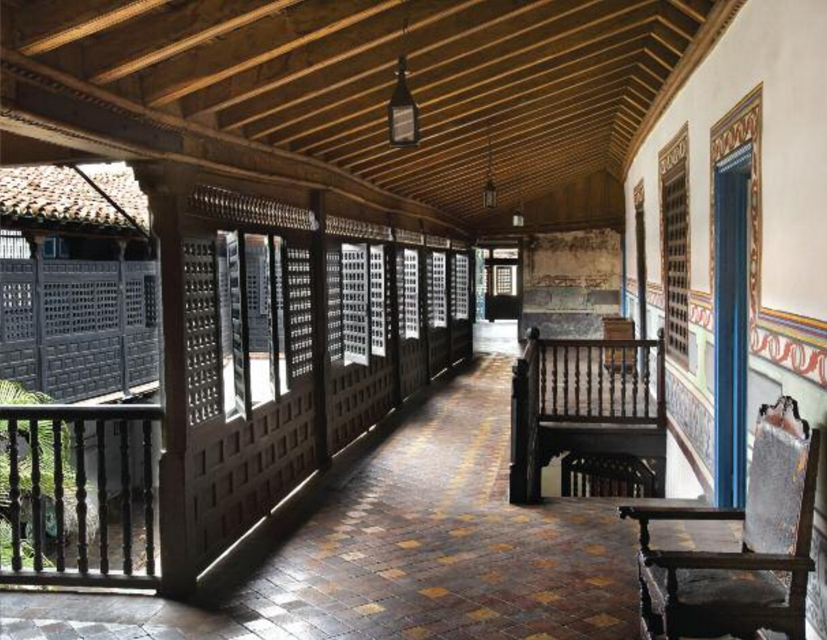
Above: Casa de Velásquez, Santiago de Cuba. Many of the gallery's screen panels are designed to pivot. They offer protection from the sun as well as allowing air to circulate. Photo by Brent Winebrenner. Courtesy of Dr. Michael Connors.
